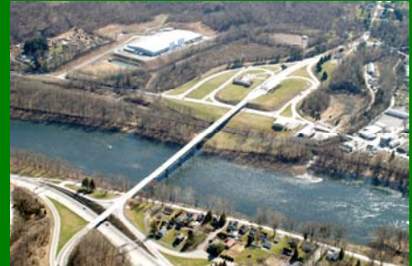
Two lane facility connecting SR 611 and Route 46
